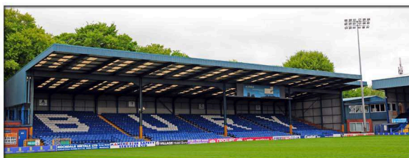
Bury FC - Stadium redevelopment
