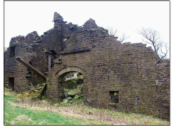
Assessing the structural integrity of derelict buildings
